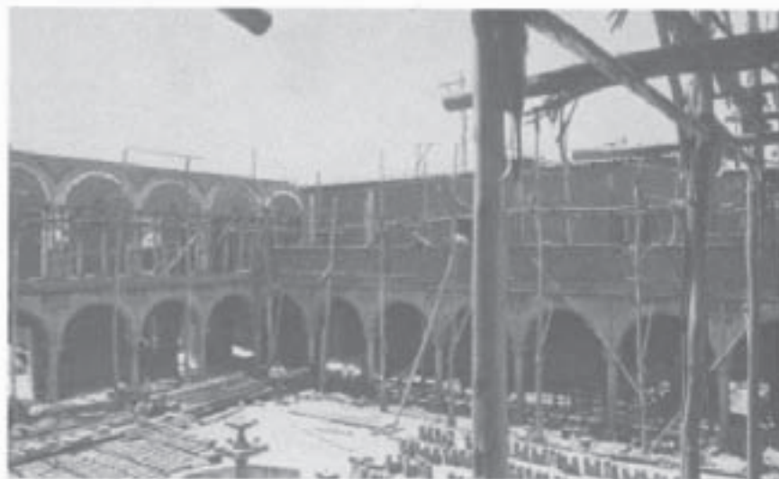
Replacement of the mud-brick wall to close one of the sides of the patio of the Palacio del Almirante in Cuzco. To enable the wall to withstand later stresses during earthquakes, it was reinforced with vertical wooden beams. Note the 'U' shape of the mud bricks which were specially made to hold the beams in place [Photo: R. Samánez Argumedo].
