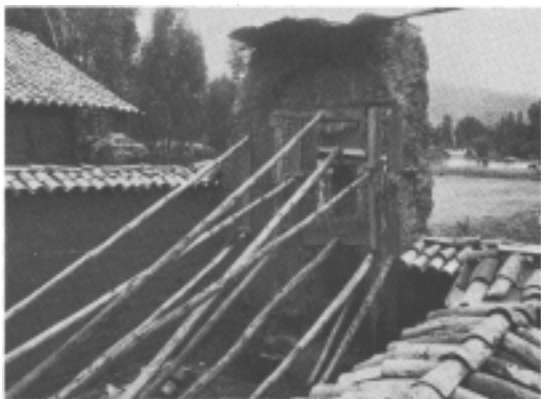
Bracing and external supports for a section of wall having vaulted niches with designs in relief and paintings of a seventeenth-century altarpiece. Lateral chapel of the church of San Jerónimo near Cuzco [Photo: R. Samáñez Argumedo].
