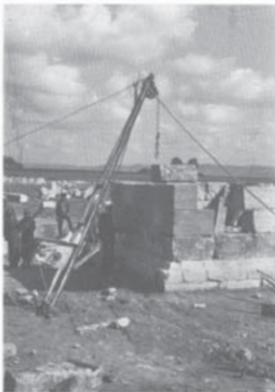
The tripod used at the Julii Mausoleum—two 'stones' made of gravel concrete (3:8) [Photo: J. Vêrité].
