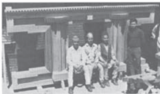
The carpentry work now complete, the window is ready for carving [Photo: Unesco/J. Sanday].
