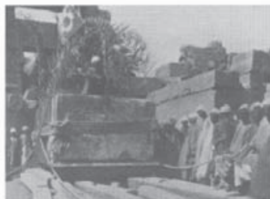
Architrave being dismantled [Photo: CNRS].
