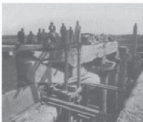
Upper portion of scaffolding, twenty metres high [Photo: CNRS].
