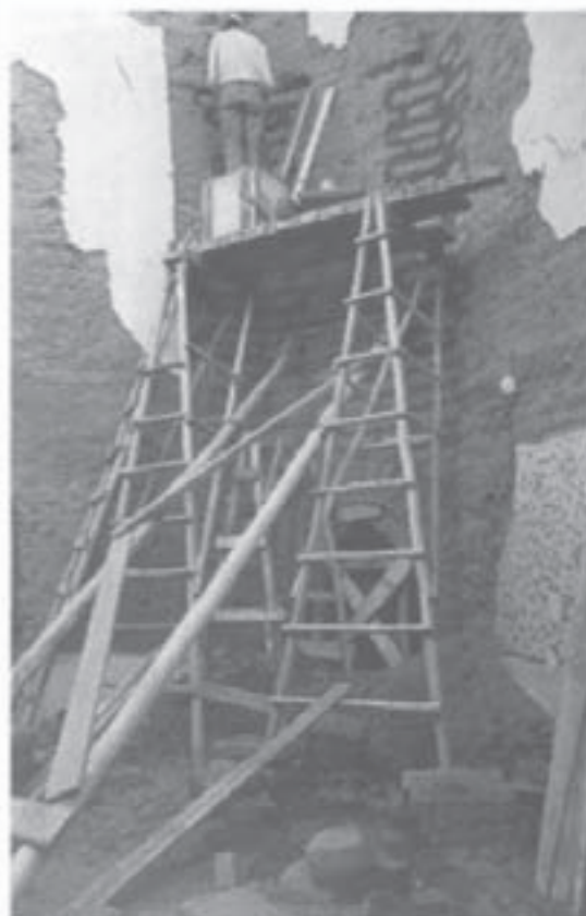
Fitting new mud bricks into a wall in order to repair vertical cracks, producing a 'seam' [Photo: R. Samáñez Argumedo].
