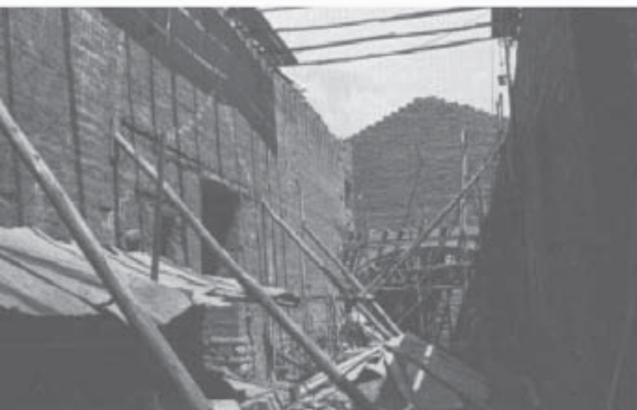
Interior of the church of the Colegio de San Bernardo during the restoration work. Placement of a special reinforced-concrete structure inside one of the mud-brick walls [Photo: R. Samánez Argumedo].
