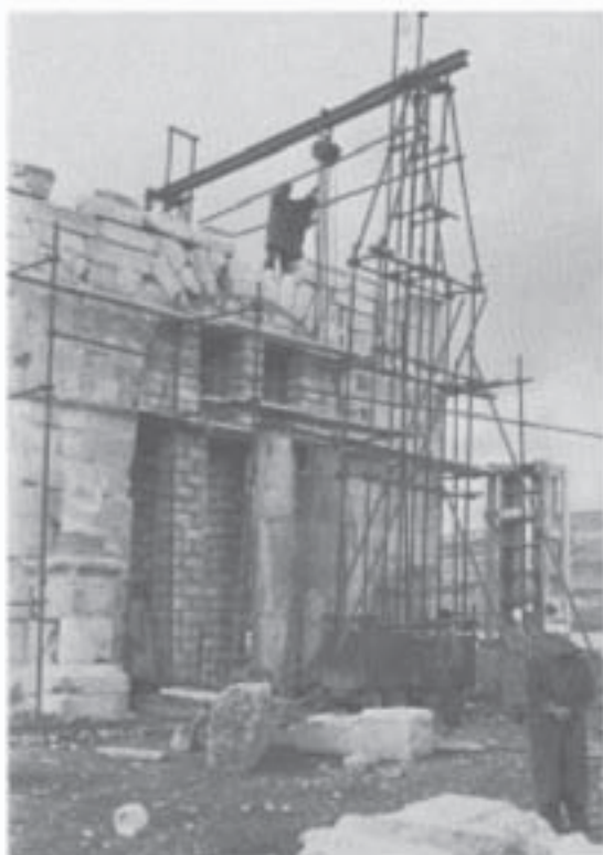
Reconstruction of columns—filling in with concrete [Photo: J. Vêrité].
