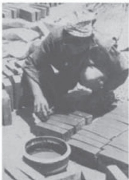
The stages of making the special telia est brick: (a) preparing the clay; (b) shaping the brick; (c) preparing the face; (d) slip glazing prior to fir- ing [Photo: Unesco/J. Sanday].
